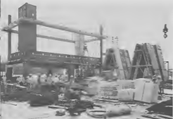
Shown here is the pre-casting of refractory slabs on the steel walls (at right) which are then installed in sections to form the furnace wall.
